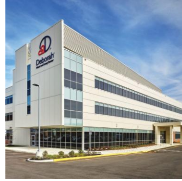
Medical Office Building, Browns Mills, NJ
